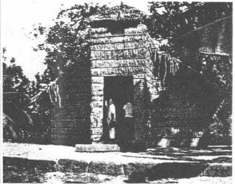
Above: When ex-Bikinians came to Kili in 1948 they built a new village under supervision, mainly using materials supplied by the Administration. This dwelling is one of thirty on Kili re-built from salvaged lumber and thatched with local pandanus. Street in foreground is sanded, rest of living area is covered with coral pebbles. Right: The Protestant church on Kili is supported by the entire island population, whose ancestors on Bikini Atoll in 1908 were the last Marshallese to be converted by American mission workers from New England.
