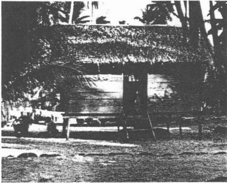
Above: When ex-Bikinians came to Kili in 1948 they built a new village under supervision, mainly using materials supplied by the Administration. This dwelling is one of thirty on Kili re-built from salvaged lumber and thatched with local pandanus. Street in foreground is sanded, rest of living area is covered with coral pebbles. Right: The Protestant church on Kili is supported by the entire island population, whose ancestors on Bikini Atoll in 1908 were the last Marshallese to be converted by American mission workers from New England.
