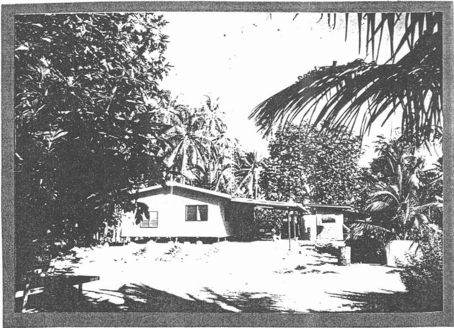
B/K/E RADIO STATION, ACROSS FROM "CHINATOWN" AREA.
